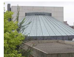
Patricia Corbett Theater, University of Cincinnati, CopperPlus roof installed in 1971
