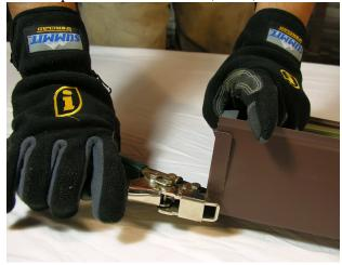
5. Next you will need to caulk the inside of the gutter that is attached to the end cap.
