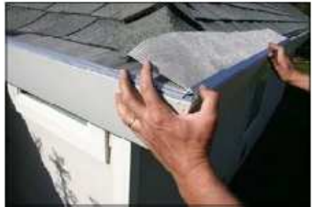
If shingles are sticking at the corner, you can use the crowbar tool very carefully to lift shingle up (N).
