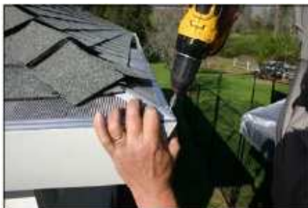
Screw down the corner fastener over the joint of both sections of Filtrate Gutter Guard.
