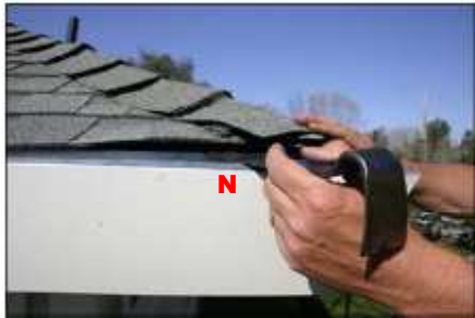
If shingles are sticking at the corner, you can use the crowbar tool very carefully to lift shingle up (N).
