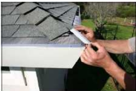
Screw down the corner fastener over the joint of both sections of Filtrate Gutter Guard.
