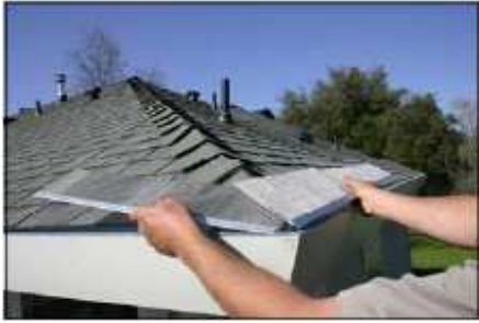
Use 2 pieces of Filtrate Gutter Guard.
