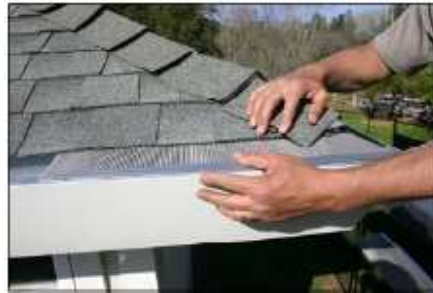
If shingles are sticking at the corner, you can use the crowbar tool very carefully to lift shingle up (N).
