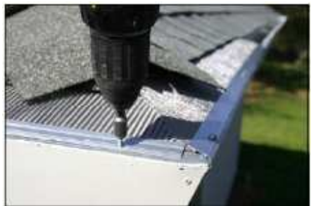
Screw both pieces to front of gutter.
