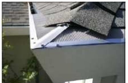
Screw both pieces to front of gutter.
