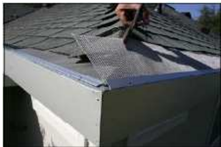
Trim other piece of Filtrate Gutter Guard.
