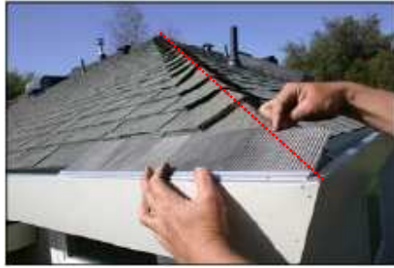
Trim Filtrate Gutter Guard at angle of roof.
