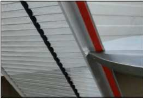
Cut the front aluminum.
