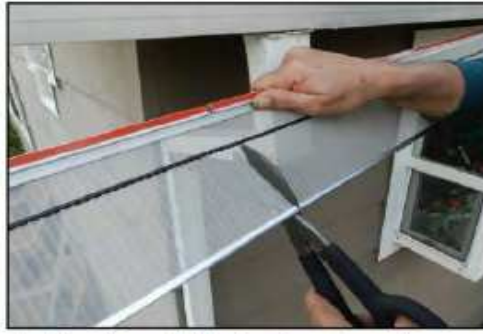
Cut the through the back and mesh.
