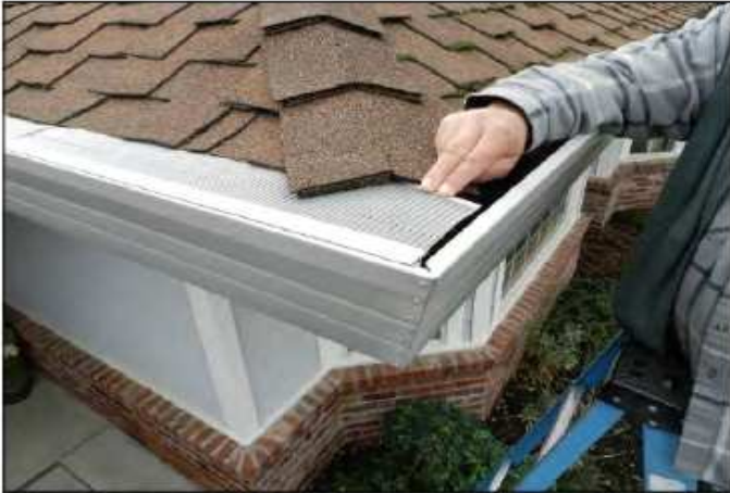
Push aluminum strip down in gutter.
