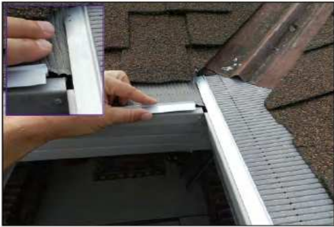
Cut aluminum so mesh hangs out.
