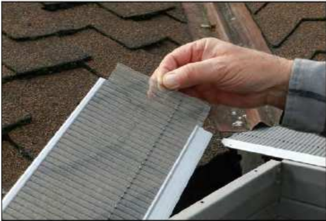
Cut aluminum so mesh hangs out.
