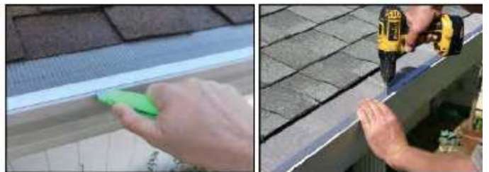
Use a sharp knife and cut tape between the gutter guard and gutter. You can apply another piece of adhesive tape to fasten it back on gutter, or you can just screw the gutter guard back down with self-tapping screws.
