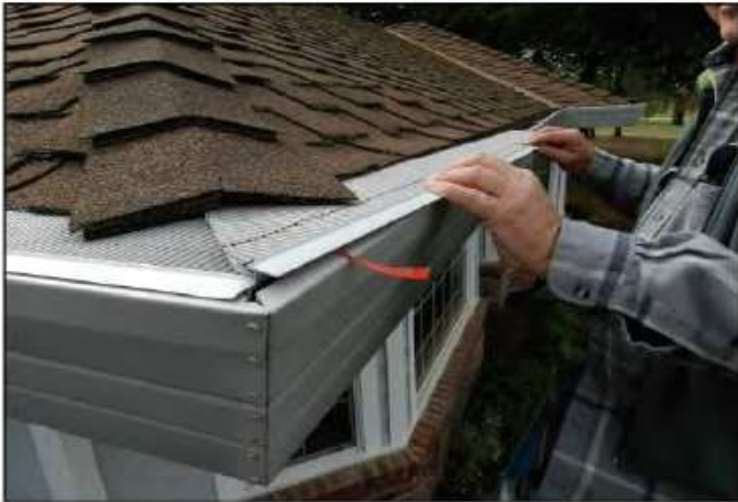
Push aluminum strip down in gutter.
