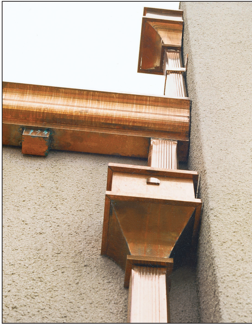
Close-up of copper gutter and ornamental conductor head. Copper Development Association
