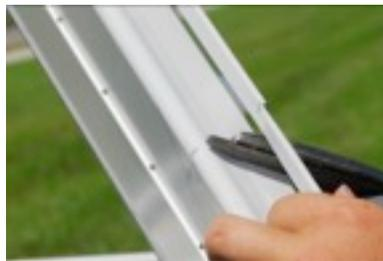
You will need to cut the underside at the same angle to create the proper fit.
