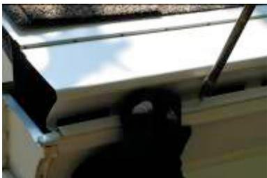
Using 2 to 3 screws per panel, fasten the panel to the gutter lip. Once the first panel is secured in place, begin positioning the next panel by starting the back edge under the tab of the first panel. This will ensure a strong over/under interlock. Push panel back, until the nose of the second panel overlaps the nose of the first panel.
