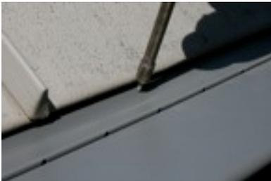
Finally, zip screw the panel to the gutter lip and down through the trim coil.
