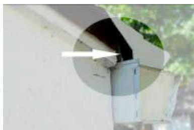
This occurs frequently with gutters that extend beyond the roof line. Even gaps this small can allow birds and small animals into the gutter system where they can quickly build nests.
