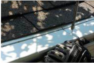
You can use an additional screw to secure the interlocking areas of the top of the panel, if desired.
