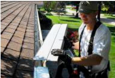
Working left to right; insert the back end of the panel under the shingles. Slide the panel into position on top of the gutter lip.
