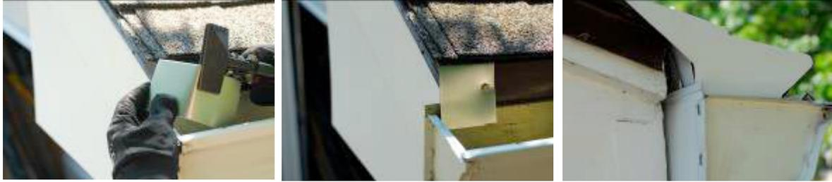
Our end caps are designed to fit six inch gutters without needing to add material. For five inch gutters, hold the end cap up to the end of the gutter and mark as needed to get the proper fitting piece.
