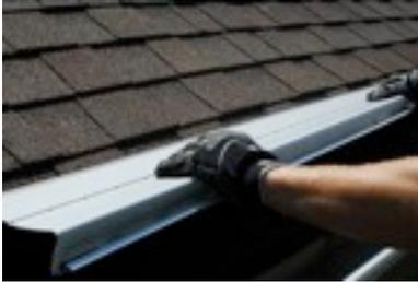
Once the shingles are loosened, adjust the panel to the appropriate roof pitch by using hand pressure or a siding break. Remember that FreeFlow should be installed with a slight 5-20 degree downward slope. It is not necessary to bend the panels if they are already within this range.
