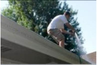
To ensure the free flow of water through the system we suggest running water into the gutter and checking the downspouts for unobstructed water flow.
