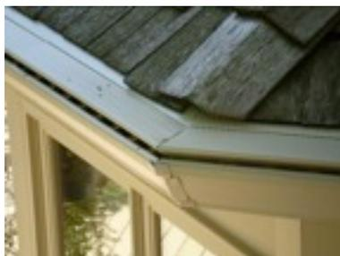
For bay windows repeat the same process, but cut the corners at a 22.5 degree angle instead of at a 45 degree angle.
