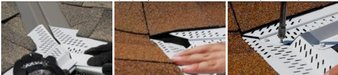
When working with valleys that have excessive water flow, use our High Flow panels in addition to the miters, for the inside corner installation.
