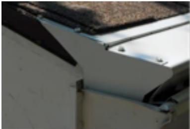
Finally, secure the end cap with two zip screws in the provided pilot holes.
