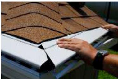
You are ready to position the second panel. Align it with the outside corner, over the top of the tab of the first panel.
