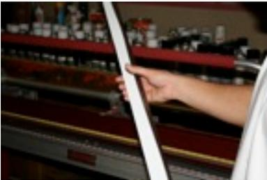
Next, measure and mark the panels approximately two inches from the hem, depending on the size of the house's gutter.
