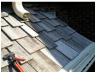
If you notice certain roofing situations that will concentrate water into heavy streams, consider ordering high water flow panels to drain the extra water.
