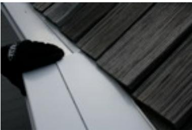
As you would in any other installation, working left to right; insert the back end of the panel under the shingles.
