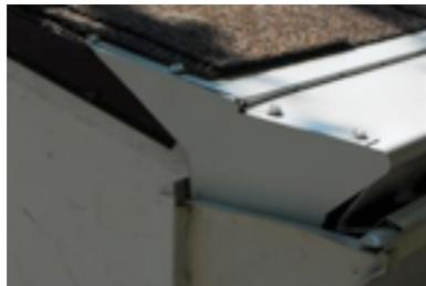
In order to ensure a properly finished end cap there can be no gaps thumb sized or larger.
