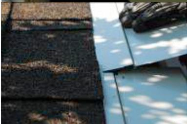
Insert the tab of panel 1 into the opening in panel 2. Secure with zip screws through the gutter lip.
