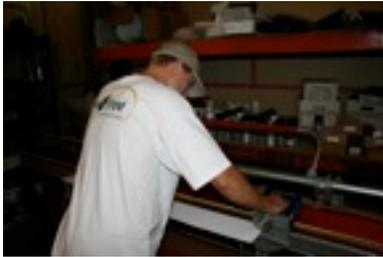
For metal and tile roofs, cut the trim coil to strips measuring ten feet by three inches.
