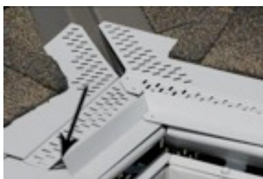
In order to install the inside miter, first mark and trim the corner panels to fit.
