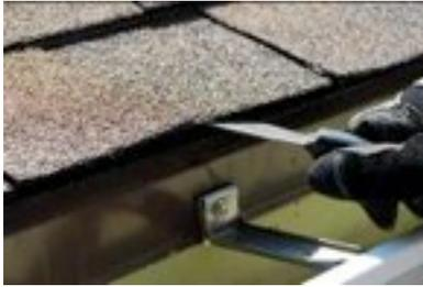
Before beginning the installation, you must determine, based on ease of installation, whether the panels will be best installed under the first row of shingles or between the starter row and the first row of shingles. Use a putty knife to loosen the shingles as needed.
