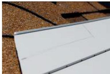
To avoid the nails in the roof crown, mark and trim the upper portion of the panel as shown.
