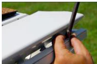
Now that the panel is custom trimmed to fit, slip it under the shingles and fasten to the gutter lip.
