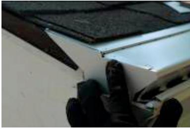
To finish, position the upper flange under the shingles and the installation flange over the cover.
